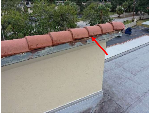
Photo 25 Building Alhambra – Roof - Overall view of coating delamination of the wood fascia.
