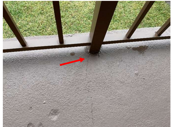
Photo 16 Building Cadiz – 2 nd Floor - Overall view of cracking in the concrete slab.
