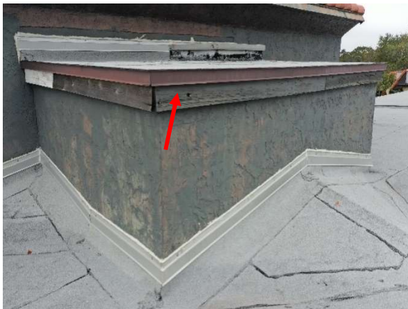
Photo 26 Building Cadiz – Roof - Overall view of deterioration of the wood fascia.
