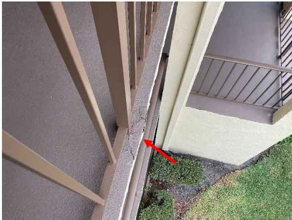
Photo 13 Building Alhambra – 3rd Floor - Overall view of spalling in the concrete slab.
