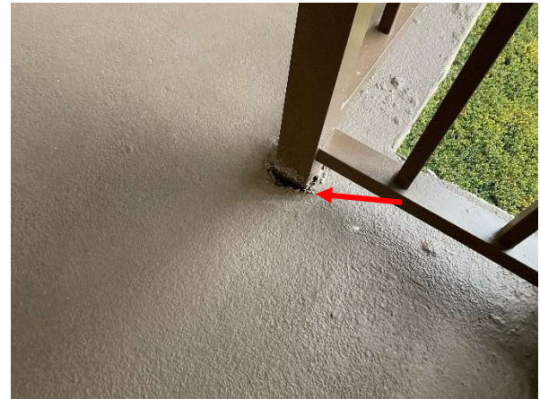
Photo 10 Building Cadiz – 3rd Floor – Overall view of railing post base not sealed to the concrete.
