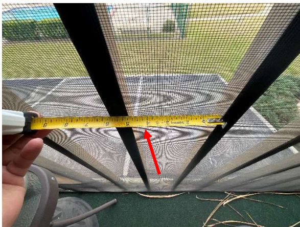
Photo 9 Building Alhambra – Unit No. 205 – Overall view of spacing between guardrail pickets greater than 4”.
