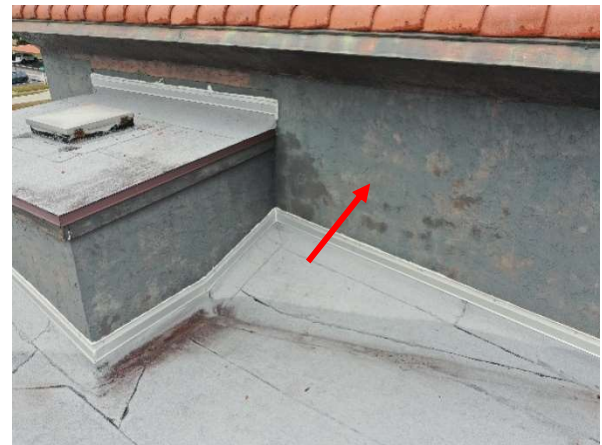
Photo 29 Building Cadiz – Roof – Overall view of exterior wall missing coating.
