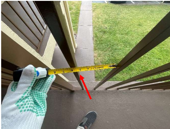
Photo 7 Building Cadiz – 2nd Floor – Overall view of spacing between guardrail pickets greater than 4”.
