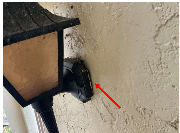
Photo 23 Building Barcelona – 3rd Floor - Overall view of wall penetration not sealed.
