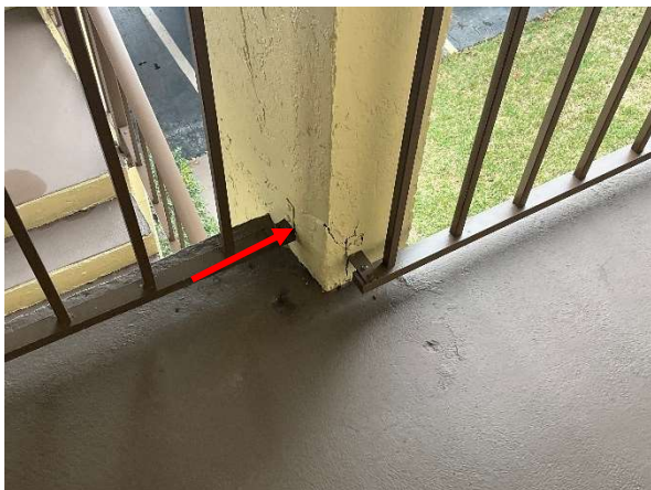
Photo 155 Building Alhambra – 3rd Floor - Overall view of spalling in the stucco cladding.
