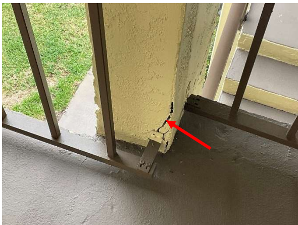
Photo 14 Building Alhambra – 3rd Floor - Overall view of spalling in the stucco cladding.
