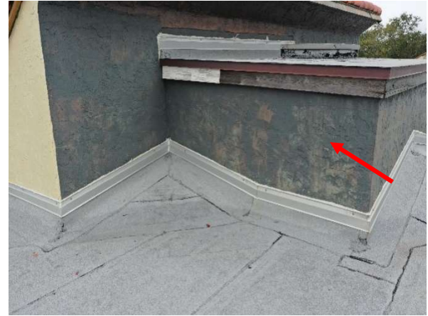
Photo 28 Building Cadiz – Roof – Overall view of exterior wall missing coating.
