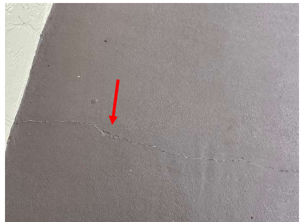
Photo 18 Building Alhambra – 2 nd Floor - Overall view of cracking in the concrete slab.
