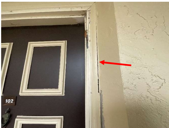
Photo 21 Building Barcelona – Unit No. 102 - Overall view of missing sealant at dissimilar material interfaces.
