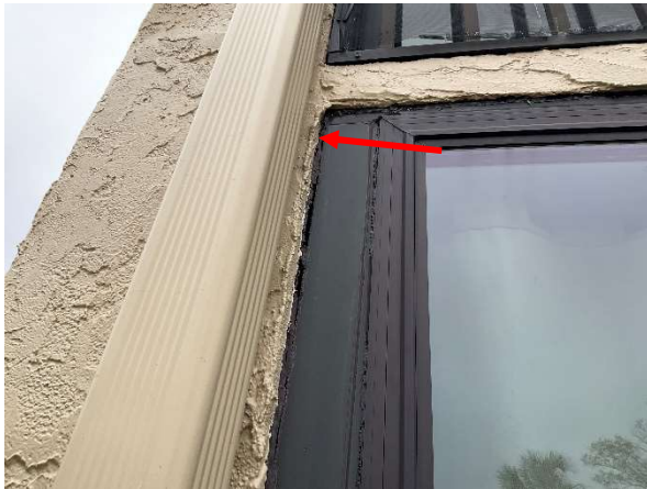
Photo 19 Building Cadiz – 1 st Floor - Overall view of deterioration and voids in the sealant joint.
