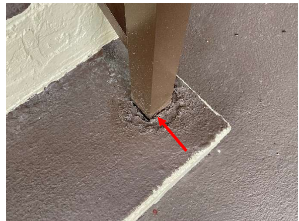
Photo 11 Building Cadiz – 1st Floor – Overall view of railing post base not sealed to the concrete.
