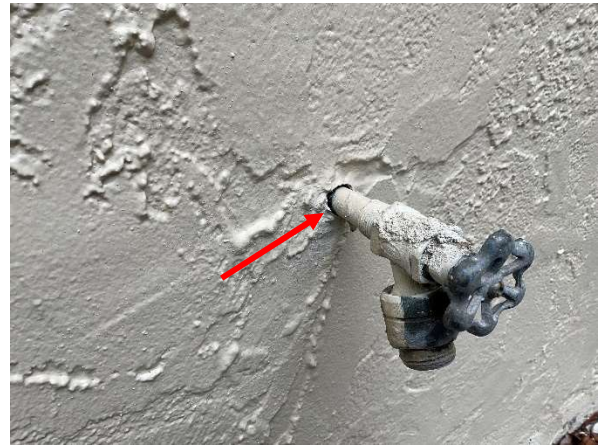
Photo 22 Building Cadiz – 1 st Floor - Overall view of wall penetration not sealed.
