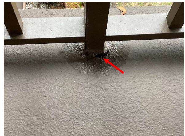
Photo 12 Building Barcelona – 3rd Floor – Overall view of railing post base not sealed to the concrete.
