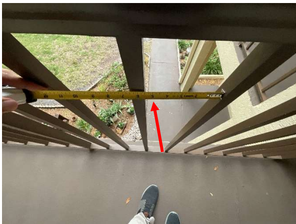
Photo 8 Building Barcelona – 2nd Floor – Overall view of spacing between guardrail pickets greater than 4”.
