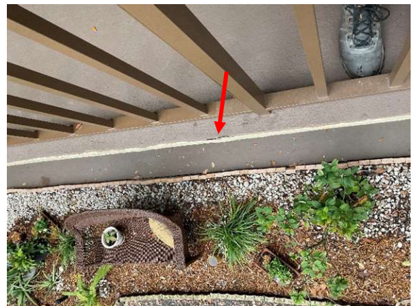
Photo 17 Building Barcelona – 2 nd Floor - Overall view of spalling in the concrete slab.
