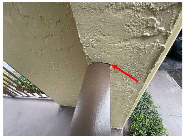
Photo 24 Building Alhambra – 2nd Floor – Overall view of missing sealant at dissimilar material interfaces.
