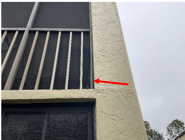
Photo 20 Building Barcelona – 2nd Floor - Overall view of missing sealant at dissimilar material interfaces.
