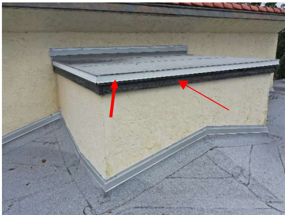
Photo 27 Building Barcelona – Roof - Overall view of deterioration of the wood fascia.
